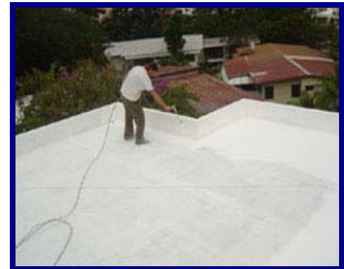
Permakote on Modified Roofing
